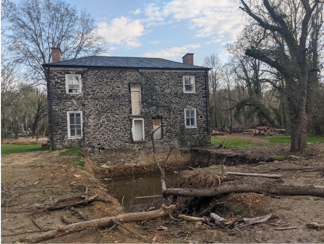
Image 8: View of north elevation (4/7/2021)
