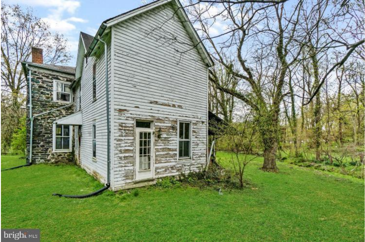
Image 6: View of north elevation (2020 listing photo)
