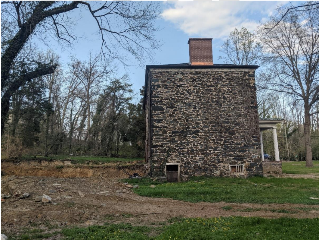
Image 11: View of west elevation (4/7/2021)
